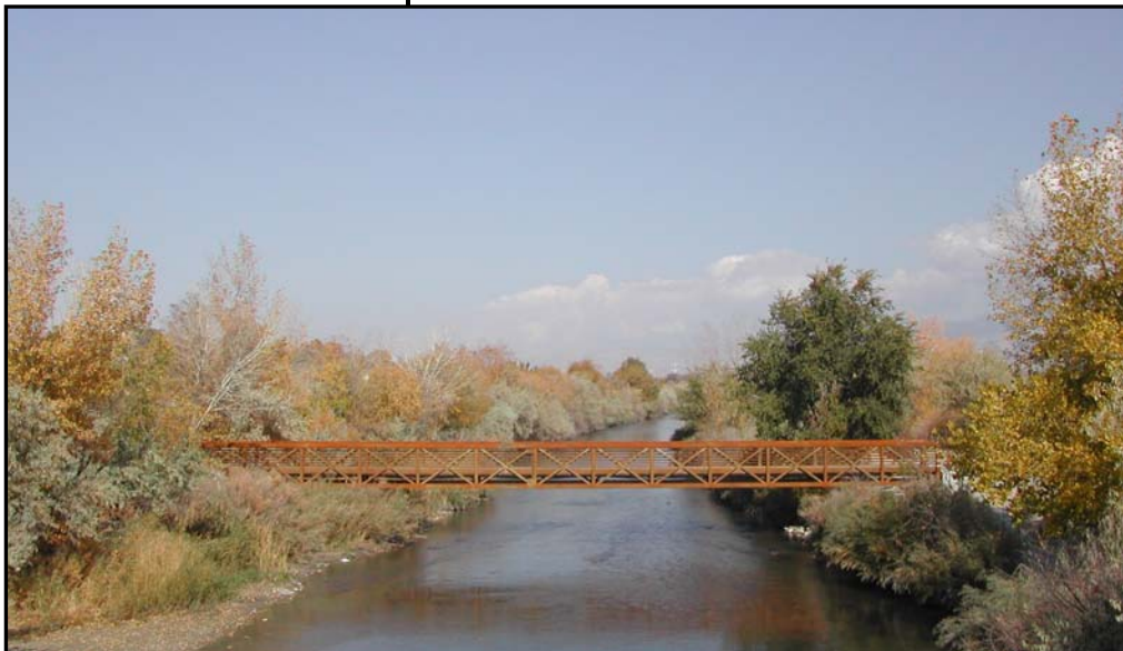
Illustration 6.4.1: Jordan River Parkway Pedestrian Bridge at Millrace Park
